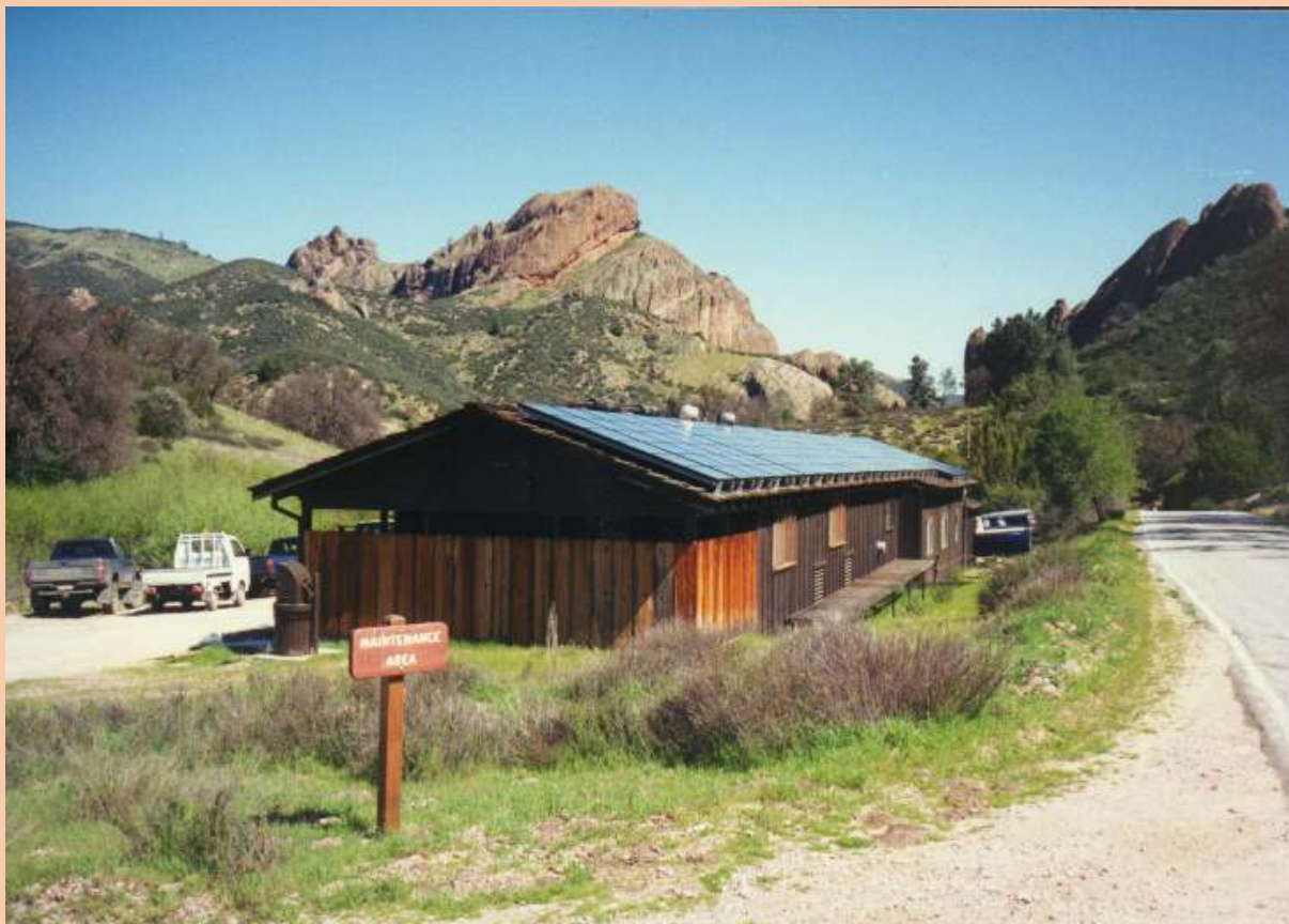
Nexgen Energy Systems installation of the original Hybrid PV power system in Pinnacles National Monument, CA
